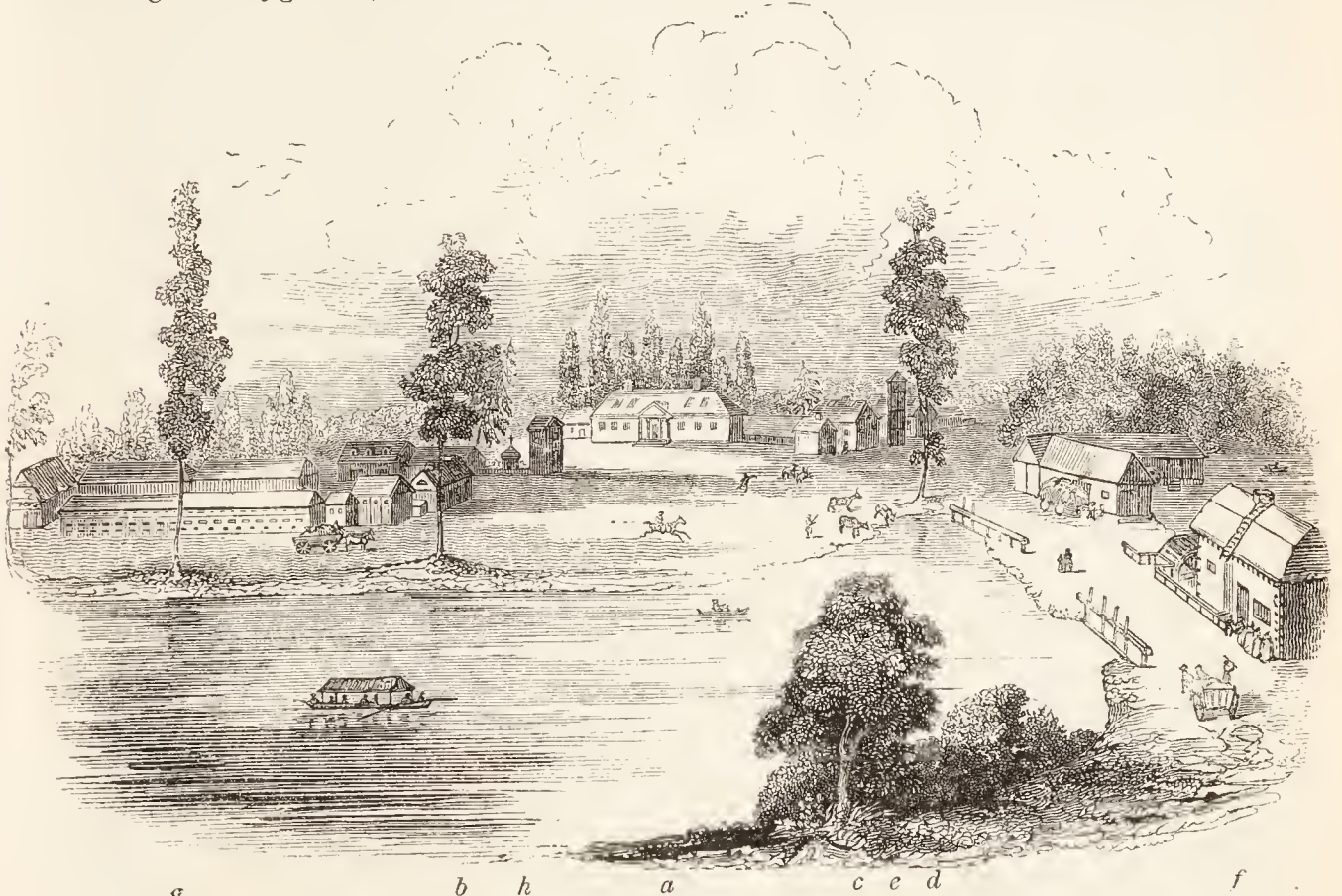
g b h a c e d f in 1832. The buildings consist of a dwelling-house ( a ), with a detached kitchen ( b ), a brewery ( c ), a distillery ( d ), a machine for raising water to supply both ( e ), a corn-mill ( f ), sheds for feeding cattle ( g ), an ice-house ( h ), in which ice is kept above ground by means of thick double walls and doors; and large barns, a threshing-machine, coach-house, stabling and all other offices, including a carpenter's shop and house, blacksmith's shop and house, bailiff's house, &c. Besides these there is a small colony of cottages for the common labourers. These cottages are generally of the kind called log houses, and, with their draw-wells attached, present the appearance of fig. 1149. The Germans who are settled in Poland, as agricul-
